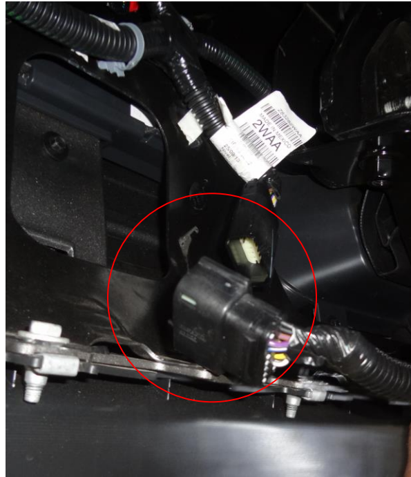
Figure 3(electrical harness disconnected)
